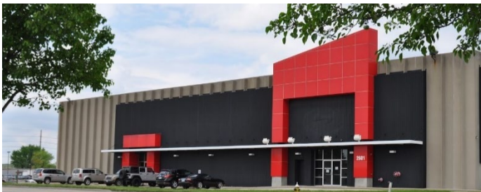
Bront Machining, Inc.'s current building on W Dorothy Lane in Dayton, Ohio
