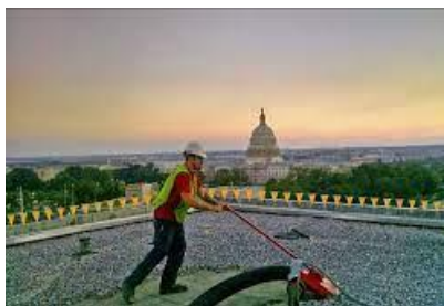
Roof Vac In Process
